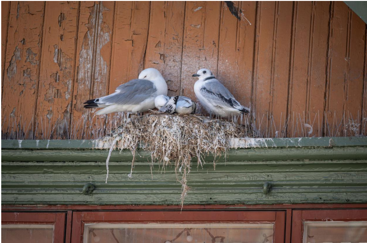
Nest directly on spikes on an historical building in Tromsø city center.
